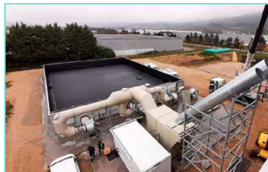
Biofilter installation in progress
