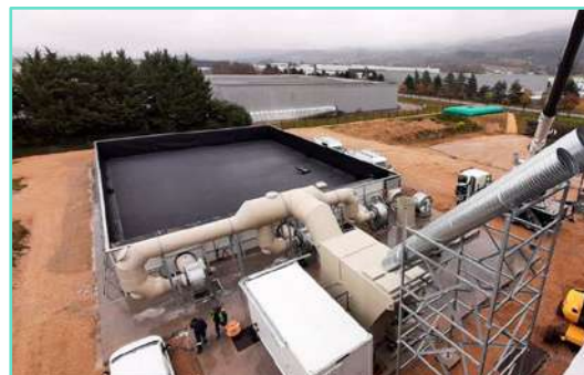
Biofilter installation in progress
